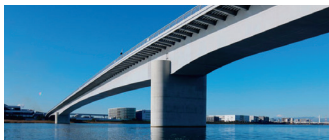
Tamagawa Sky Bridge
